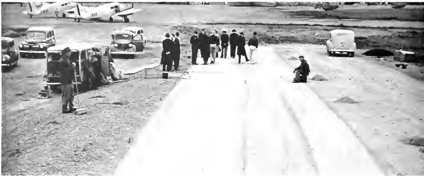
Army engineers inspect runway test pavement at Stockton field. Electric recording equipment for measuring subgrade pressure and pavement deflection under heavy wheel loads is mounted in station wagon at left
